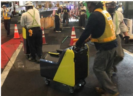
Hydrogen fuel cell generator can be easily carried
