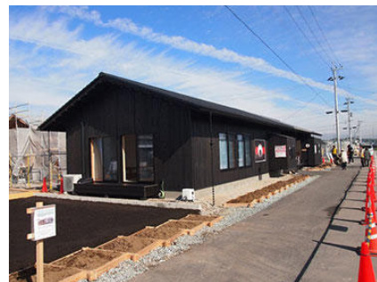
"Minna no Ie" (Home-for-All) at Techno Temporary Housing Complex in Mashiki Town
